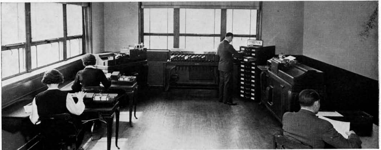
A Well-Planned Installation
